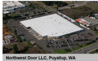
Northwest Door LLC, Puyallup, WA
